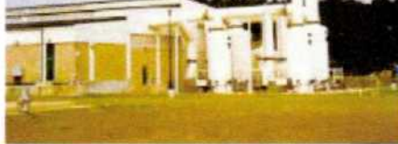
Exhaust air from the preliminary treatment building is routed through wet chemical scrubbers to remove odorous gases.
